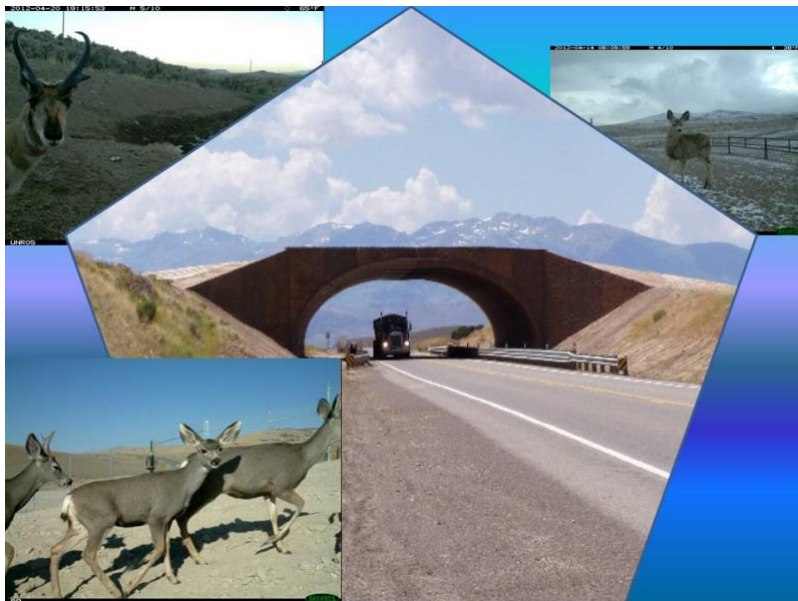
Highway 93 - Big Game Overpass – Monitoring Research
